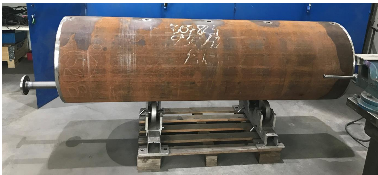
Figure 4.8: Vessel base body under construction
