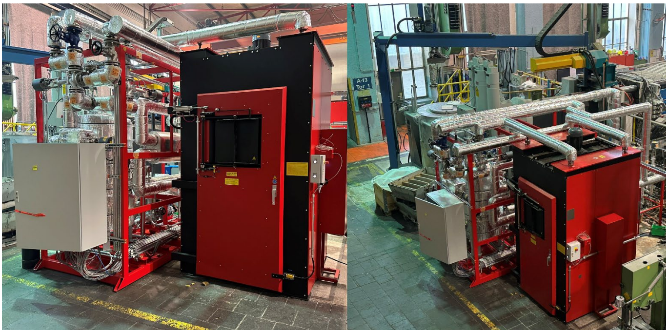
Figure 35: Installation of the combined aluminum pre-heating and annealing furnace the Green Foundry 4.0 demo factory at AIT LKR Ranshofen.
