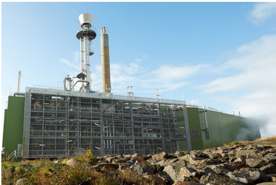
Figure 14: A 20 MW gasification project was successfully demonstrating the technological viability in Gothenburg ( The GoBiGas Project )
