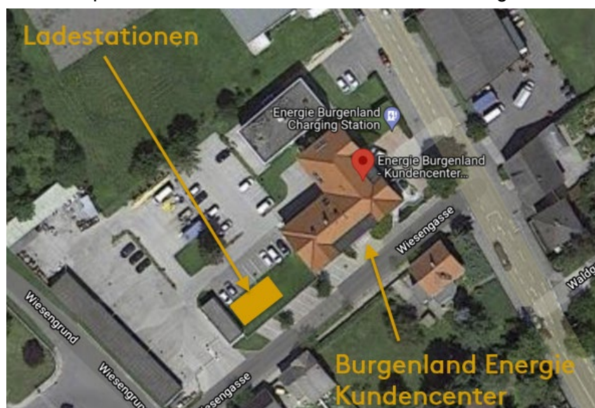
Figure 77: Overview Fuhrpark Burgenland Energie
